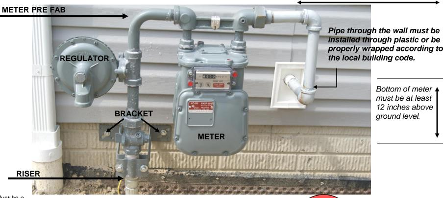
Bottom of meter must be at least 12 inches above ground level.
